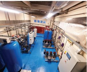
By installing the new treatment process site were able to stop the use of both HCl and Caustic in the treatment process as the need for chemicals was removed.
