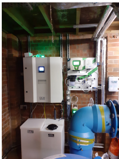
T15-30 LC Genox unit with brine tank and Neuthrox tank. Micro water softener and carbon filter. Two Prisma dosing pumps and Centurio chlorine monitor.
