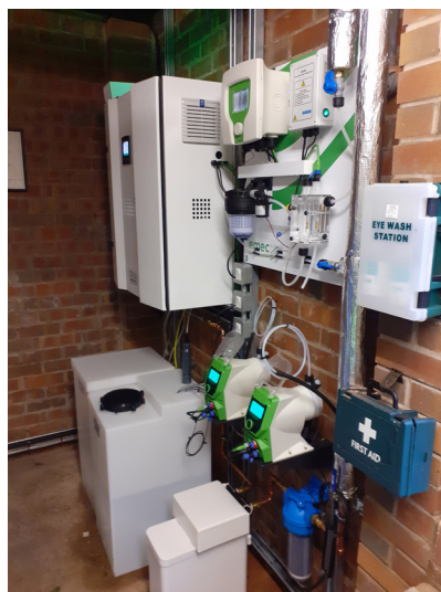
T15-30 LC Genox unit with brine tank and Neuthrox tank. Micro water softener and carbon filter. Two Prisma dosing pumps and Centurio chlorine monitor.
