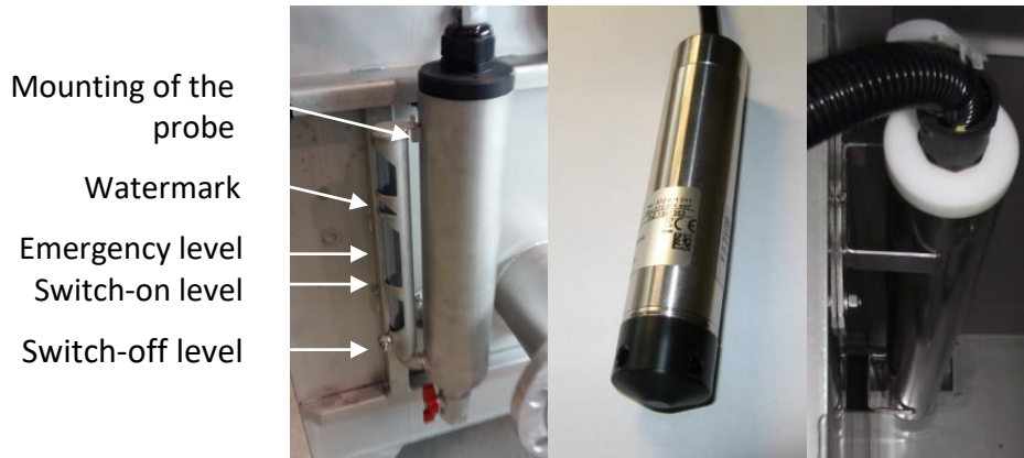
Fig. 19 Pressure probe (inlet and sludge tank)
